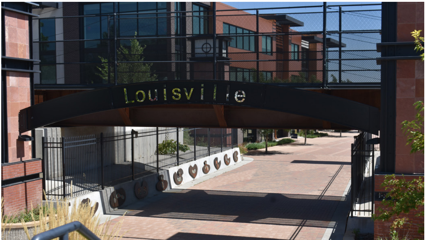
Louisville Bridge Source: DesignWorkshop
