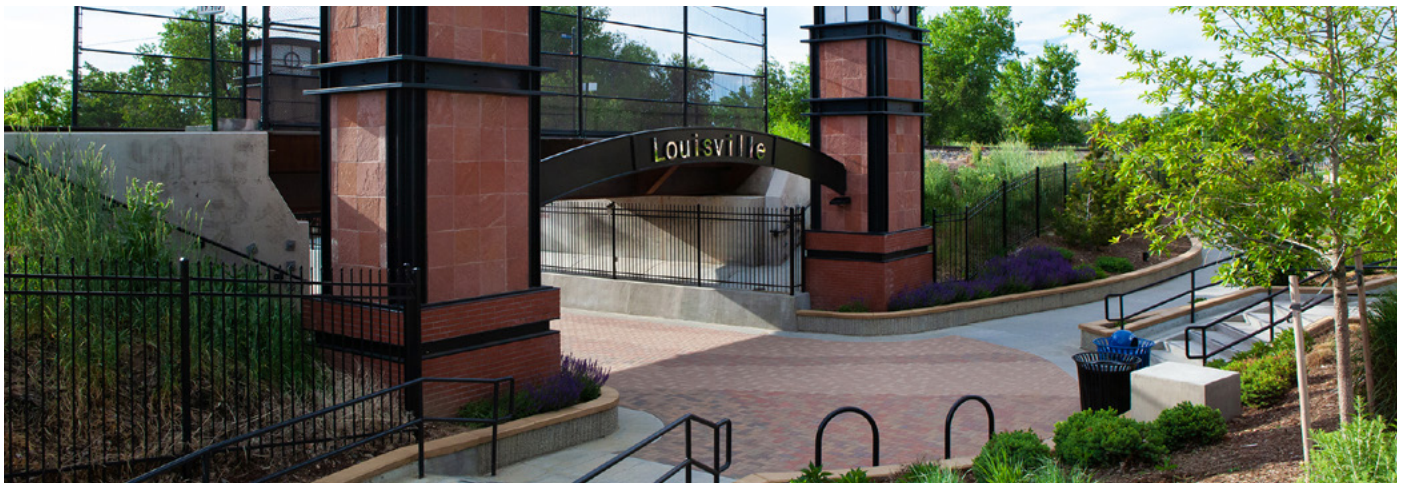
South Street Underpass Source: City of Louisville
