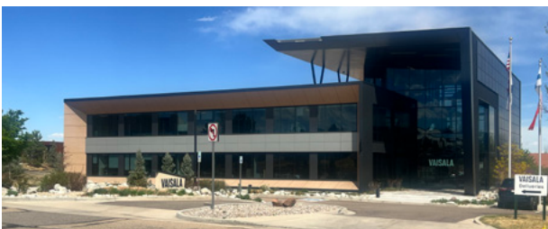
Colorado Technology Center Office Building Source: City of Louisville
