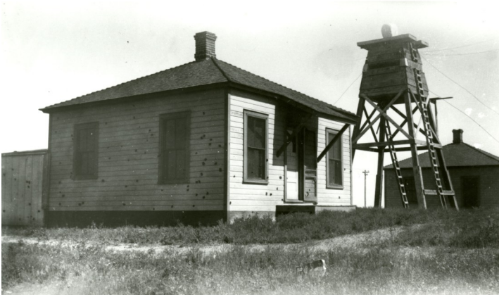
House at the Hecla mine property riddled with bullets after the shooting on April 27, 1914.
