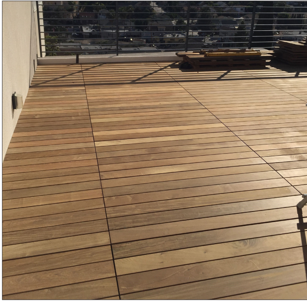
WOOD PLANK PAVER TILE DECK
